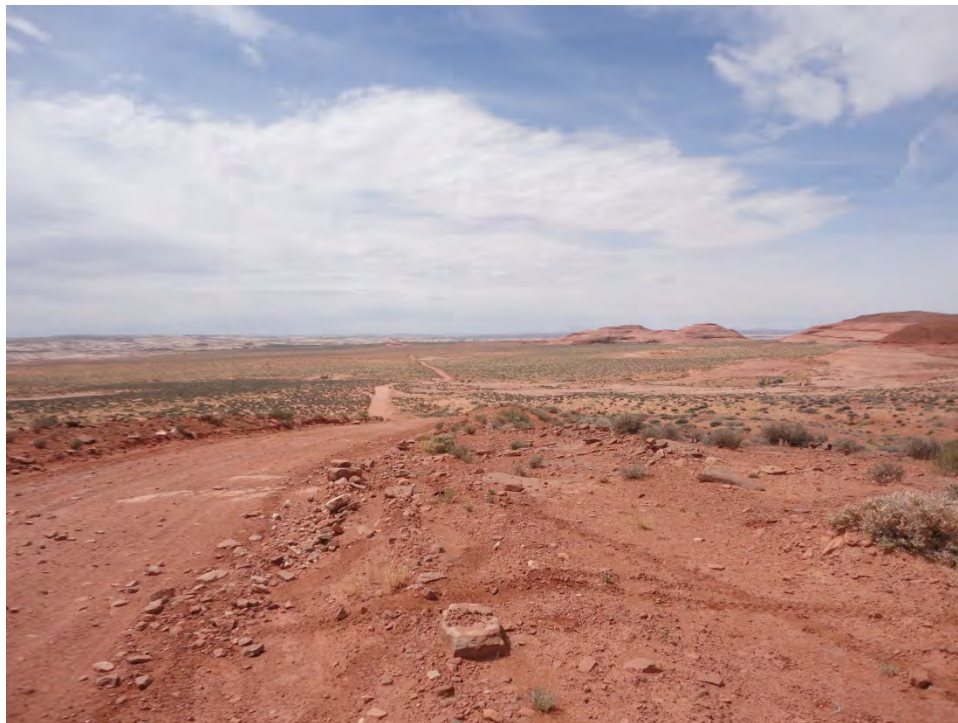
Figure 5-1. Photograph to the Southwest along Ten Mile Point Road Accessing the Northeast Corner of the Property and Historical Quintana Fed 1-1 Well in the Distance (taken 25 April 2012)
